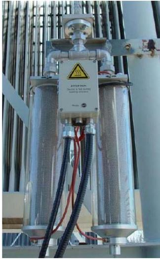
Fig. 3: Photo of MTrab<sup>®</sup>, maintenance-free dehydrating breather
